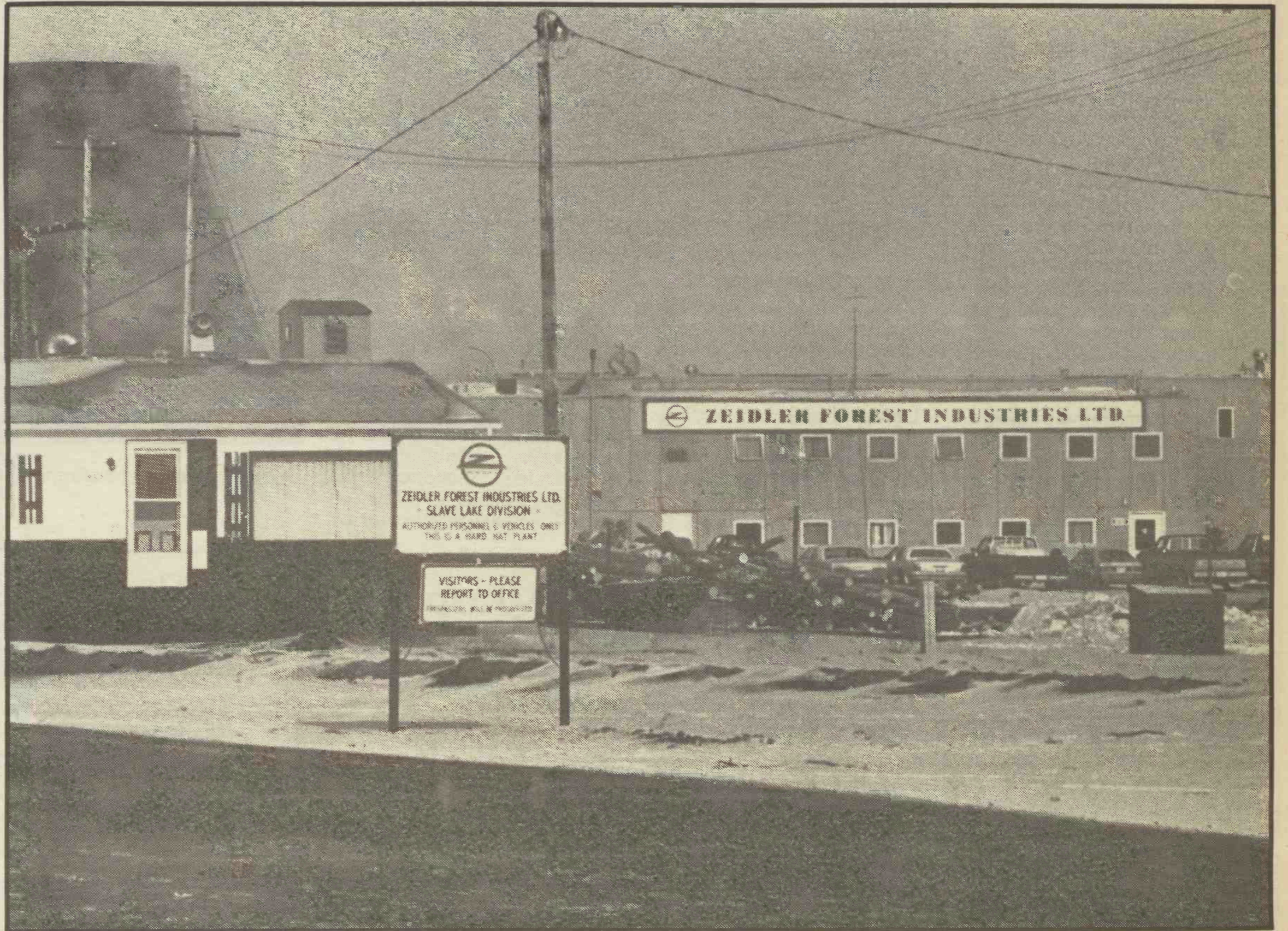
The entrance to the plant
