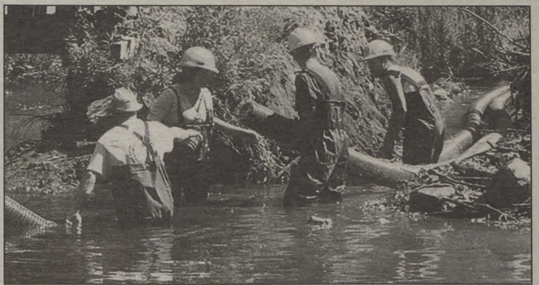
Members of the Algonquin of Pikwakanagan Earthwalkers Stewardship Ranger Team construct a beaver baffle, a device that controls water levels to provide a suitable habitat for beavers while eliminating the possibility of flooding to the benefit of landowners. The project was just one of many completed by the team as part of the eight-week Earthwalkers summer work program designed to give youth a chance to learn more about managing their natural environment.
