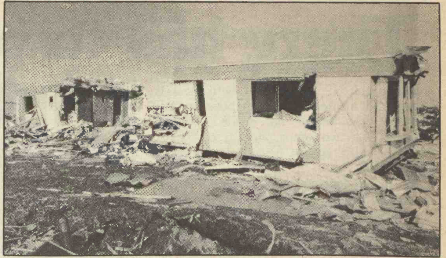
TORNADO DEVASTATION AT EVERGREEN TRAILER PARK ...trailer cut in half
